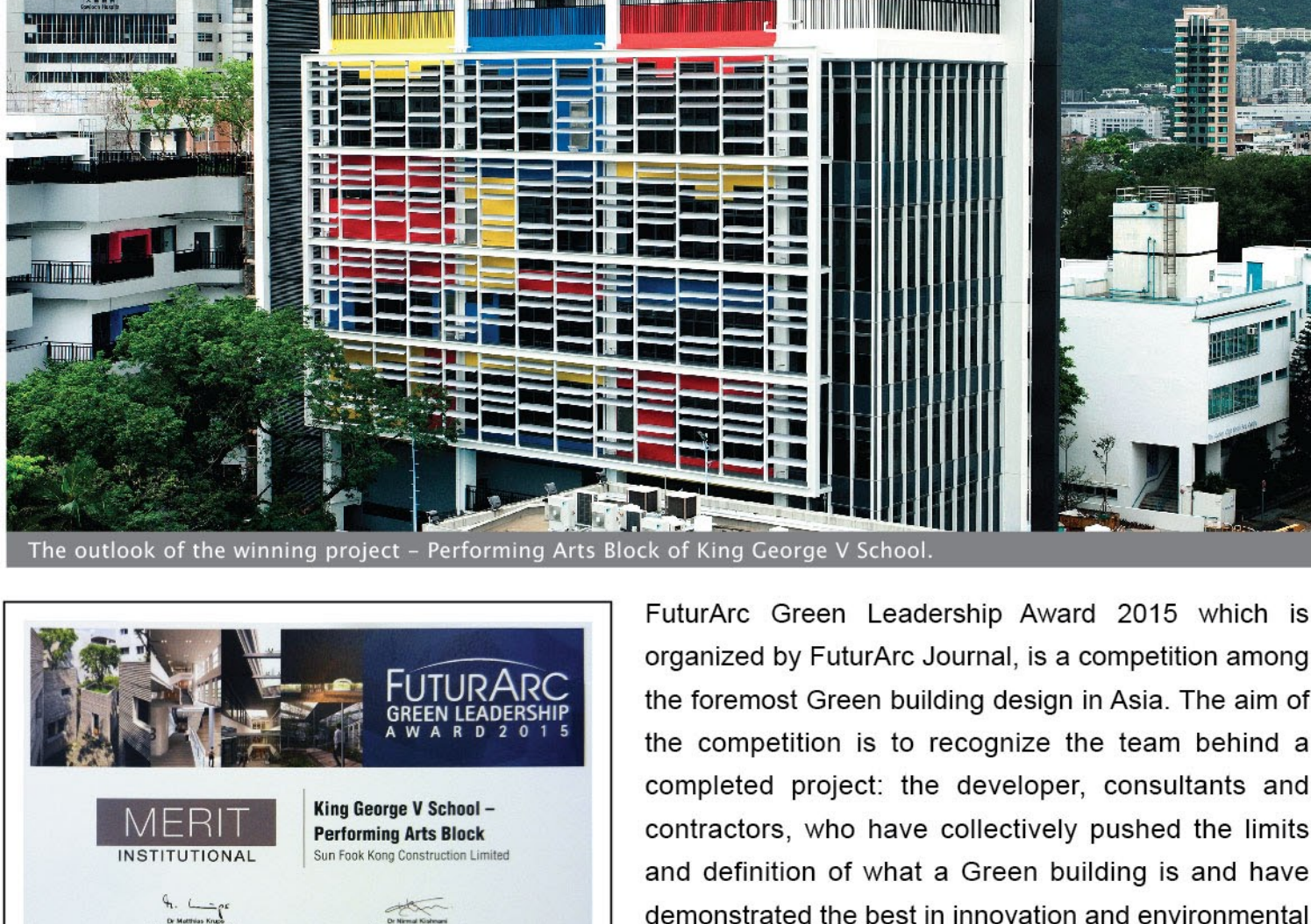
The outlook of the winning project – Performing Arts Block of King George V School.
