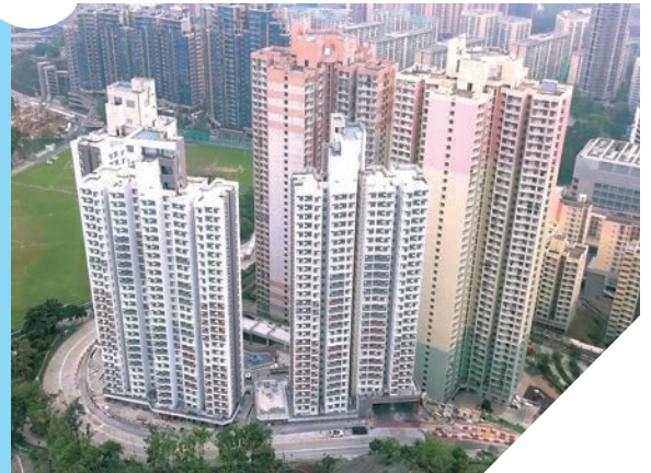
Construction of Home Ownership Scheme Development at Sheung Lok Street, Homantin 位於何文田常樂街 興建居屋發展項目 ▶
